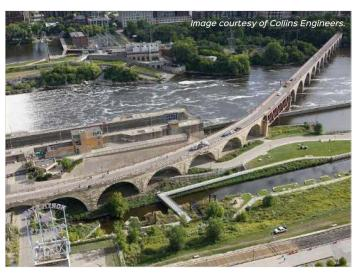
Collins Engineers used iTwin Capture Modeler to generate a high-fidelity 3D model from 13,000 drone-captured images, improving quantity and quality of data collection.
