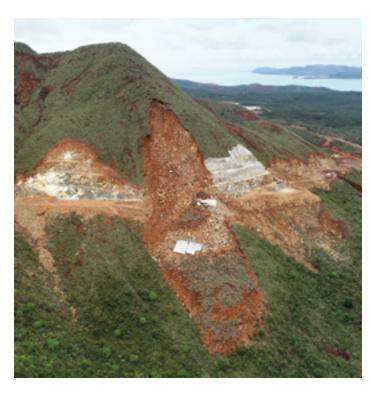
When construction of a 2.2-kilometer critical access road in New Caledonia was halted due to a landslide, engineering and construction manager Hatch initiated a comprehensive stability assessment of the area, designing a remediation plan and validating continued construction along the planned alignment. Faced with technical, coordination, and site challenges, Hatch needed a collaborative digital geotechnical solution to avoid a costly and environmentally damaging alternative realignment.
