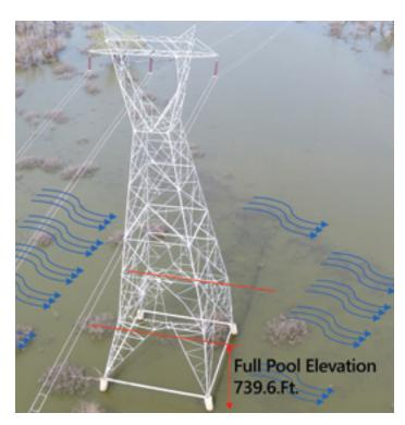
During a regular inspection, the team learned that a critical 161-kilovolt overhead transmission tower had been damaged during a recent flood. This particular line was serving power to several area hospitals that were at full capacity during the pandemic. Loss of power would have been catastrophic to the area. Exo was tasked with conducting a survey of the tower to assess its condition. However, the line needed to remain energized, requiring the team to find a safe but still efficient workflow.
