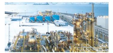
This refining and chemical integration project has an oil refining capacity of 16 million tons per year and produces paraxylene and ethylene cracking, as well as hydrogen and methane. The plant includes a refrigeration box and internal equipment that together weigh a total of about 640 tons. To consider the structural integrity during operating, lifting, and transportation conditions, the project team needed comprehensive structural design and analysis technology.
